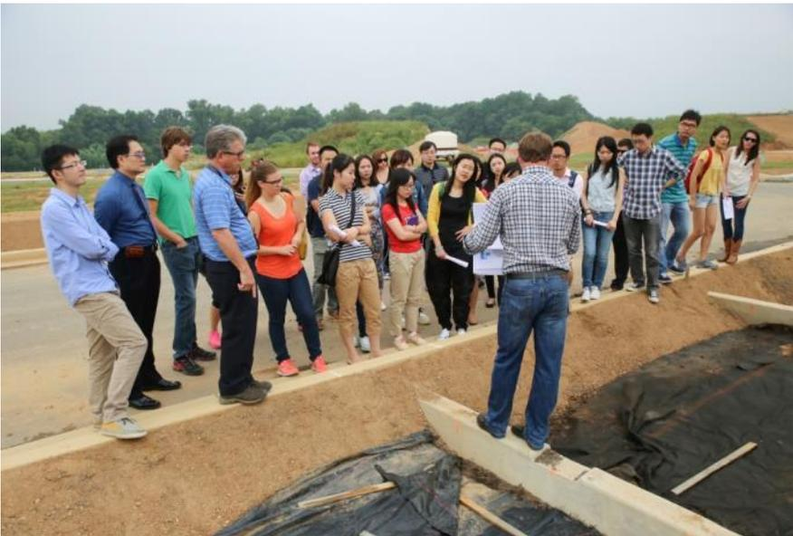
Bobby Zeiller, VP of SunBrook, hosts a comprehensive tour of Crown Farm. Here, Bobby, shows students how a bio swale is put together to mitigate stormwater run-off.
