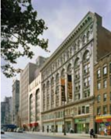
Manhattan Campus Facade After
