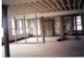
Typical Conditions Before
